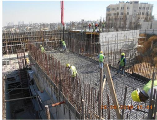
Casting water well roof slab in block III, August 2019
