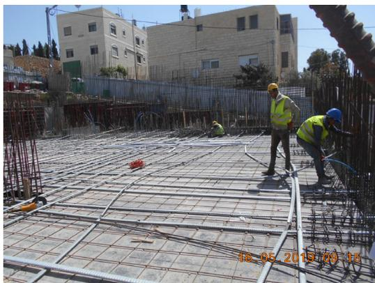
Post tension slab works in Basement -1 Block 1,
